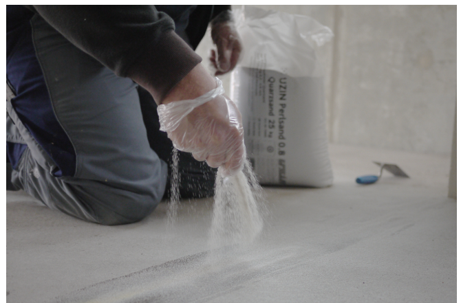
Smoothed UZIN KR 516 must be sanded with UZIN Fine Sand while fresh.
